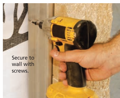
Stack units into H-Channel, secure to opposite side with H-Channel and repeat.
