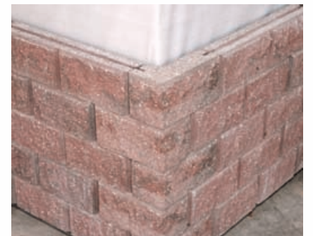
Fit H-Channel in grooves of stacked block with rubber hammer.
