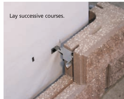
Level and adjust as you build.
